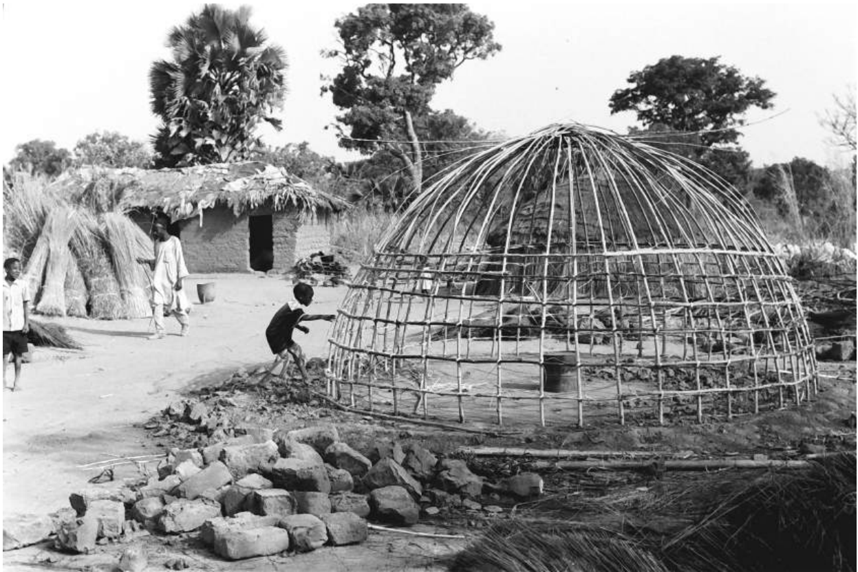
New hut under construction
